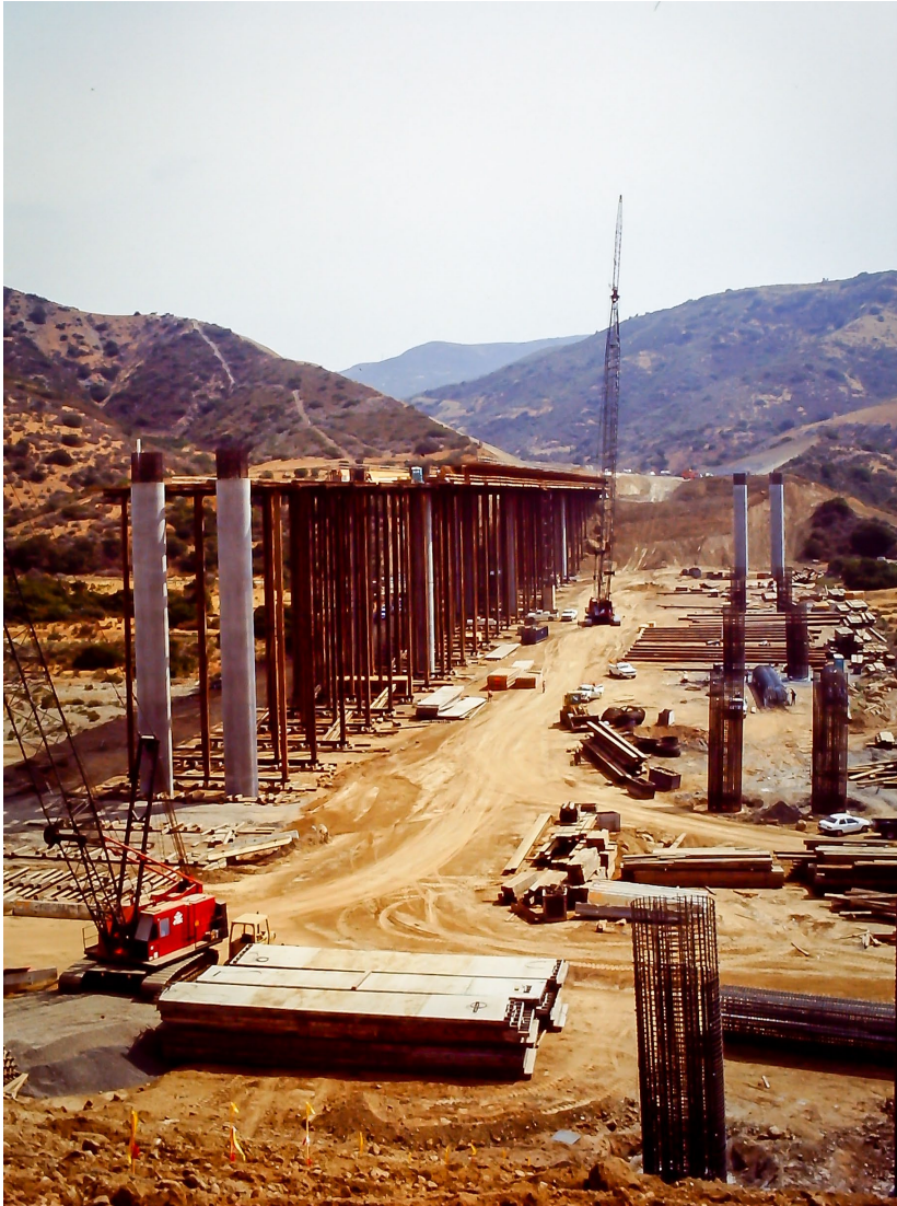
241 Toll Road — Santiago Bridge
