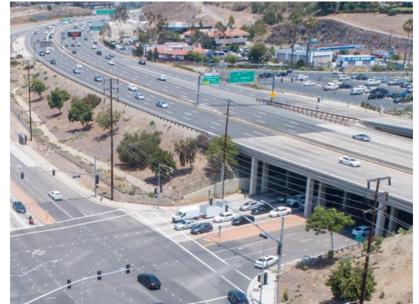
New Bridge over Lincoln Avenue
